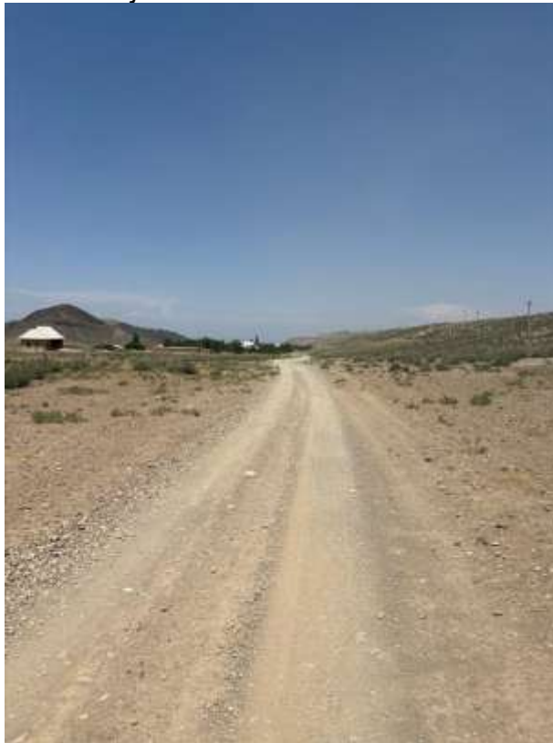
Reservoir construction site
