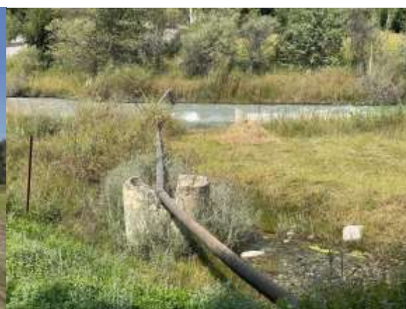
Existing pumping station
