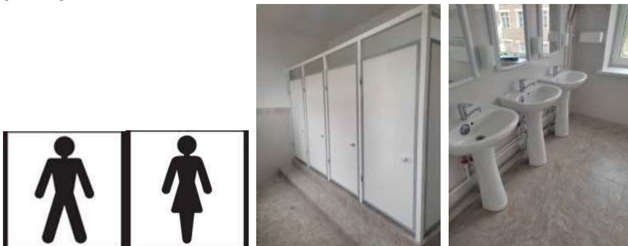
Figure 19. Example works on the subproject sites – Interior work
