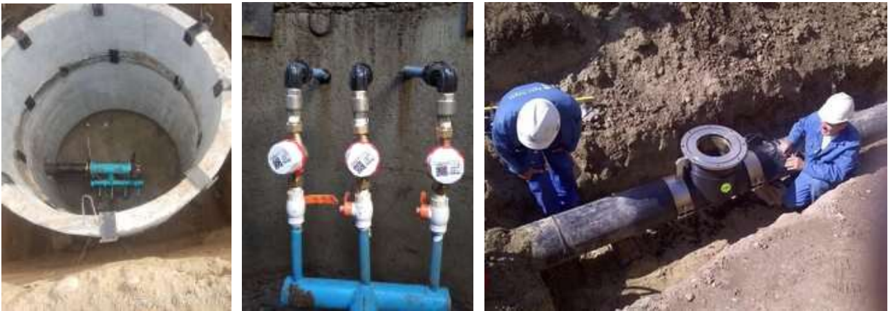
Figure 14. Example works on the subproject sites – Distribution networks
