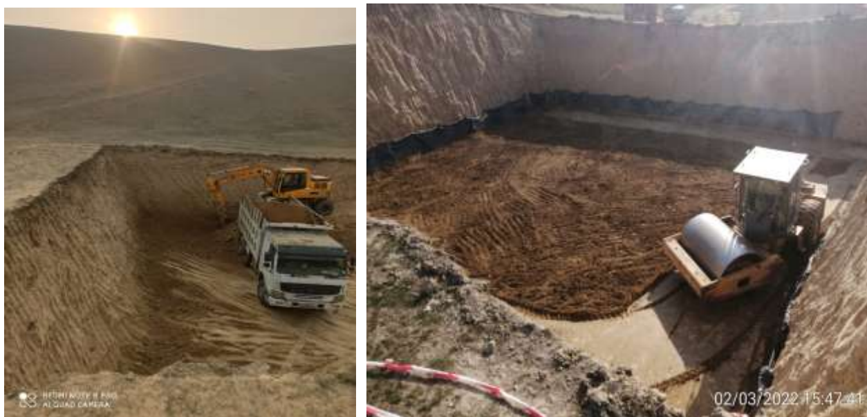
Figure 10: Example works on the subproject sites - Trench cross-section, depth of excavations, is regulated by the project
