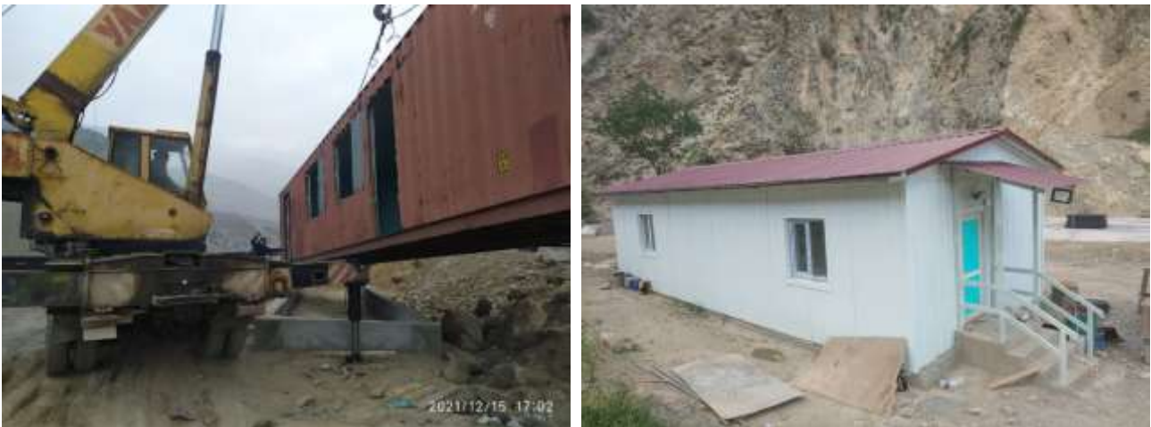
Figure 15. Example works on the subproject sites – Buildings and Structures
