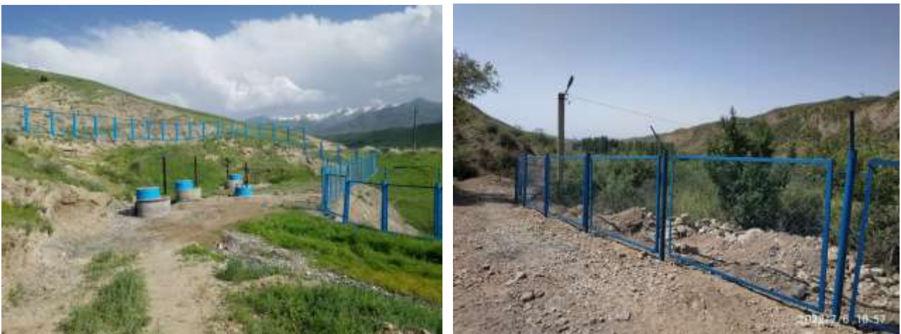
Figure 16. Example works on the subproject sites – Fences
