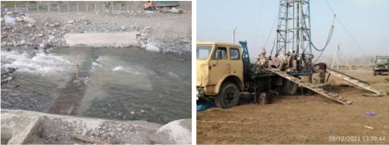
Figure 11. Example works on the subproject sites – opensource and groundwater intakes
