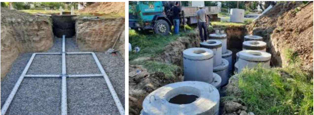
Figure 18. Example works on the subproject sites – Septic tank construction
