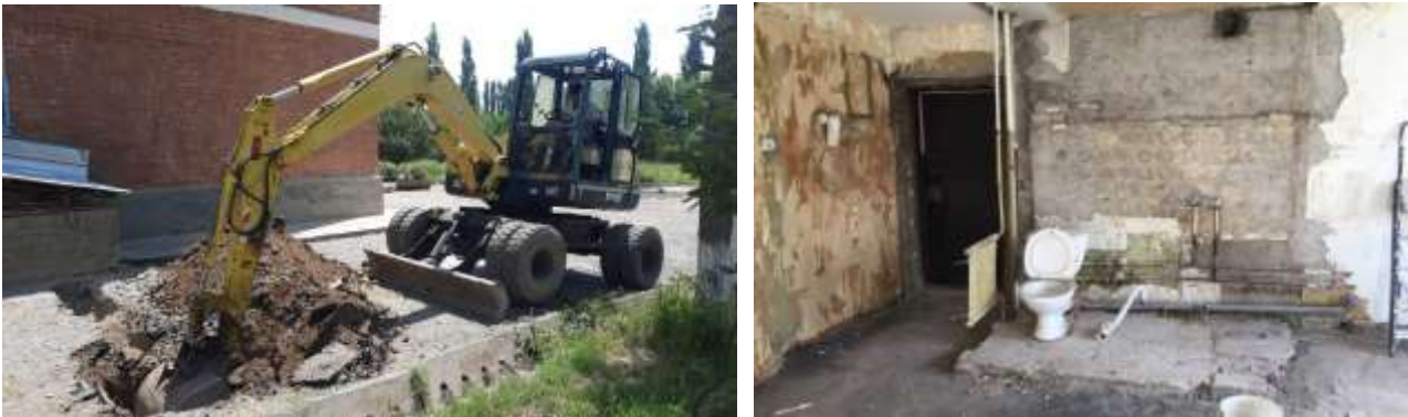
Figure 17. Example works on the subproject sites – Disassembling works
