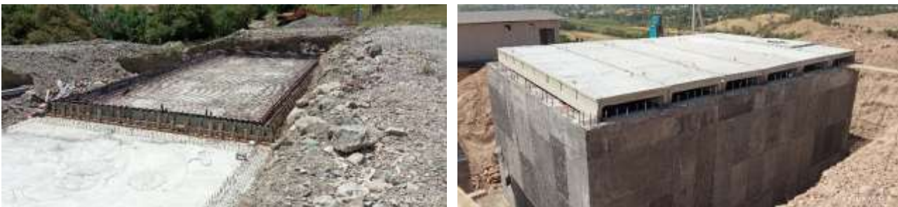
Figure 13. Example works on the subproject sites – concrete works – water tanks
